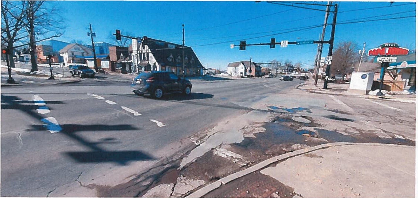
From the northeast corner looking southwest
