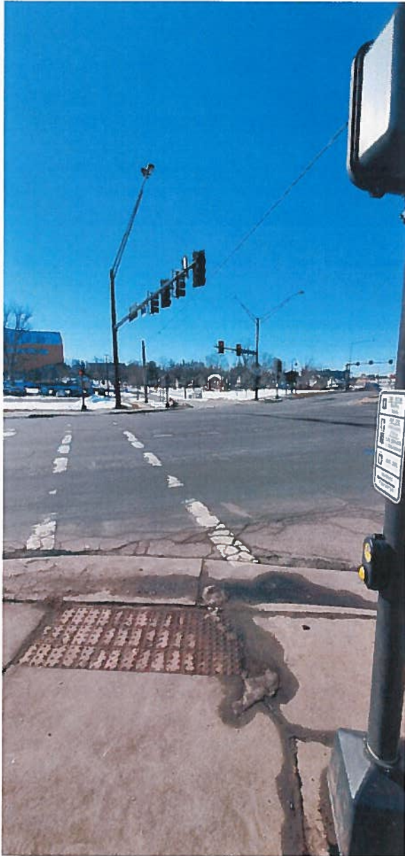
From the north to the south across East Main
