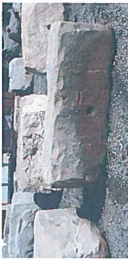
Sandstone blocks to form retaining wall to games/ event area
