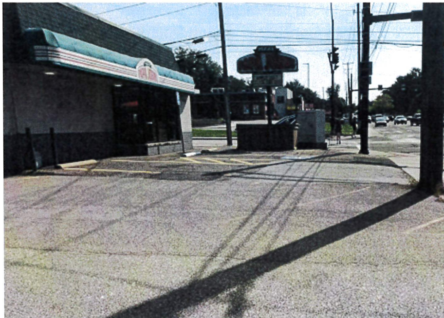
Photograph 2 – View from near station 116+80 facing in an easterly direction showing the Parcel 8T area; the Papa John's sign is shown on the right of way plans to be a "do not disturb" item
