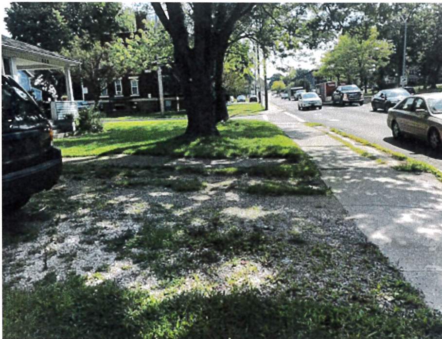
Photograph 2 – View from near station 124+50 facing in an easterly direction showing the Parcel 13T area; the two trees along the E. Main Street frontage are shown on the right of way plans to be “do not disturb” items
