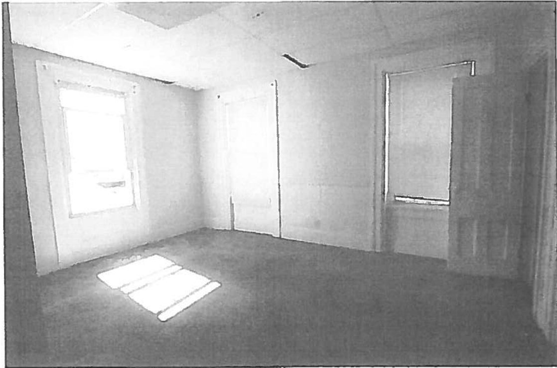
Note Intact Window Paneling...Typical
