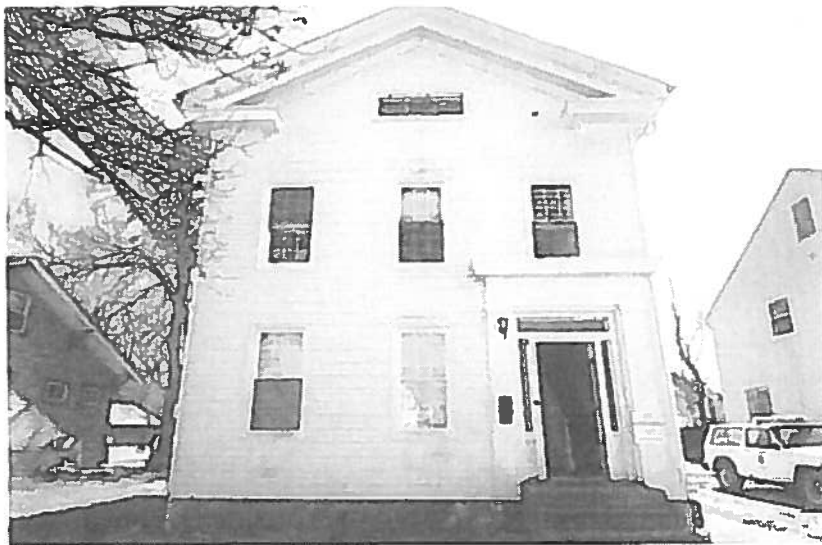
View of North Elevation/Front
