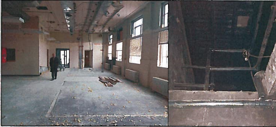
John Flynn Courthouse Renovation
