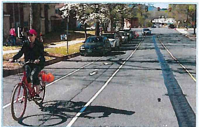
Provide dedicated facility for uphill bicyclists: A two-lane street with parking on both sides is redesigned with a climbing bike lane. Note the centerline had to be covered, which added an extra level of complexity to the demonstration.
