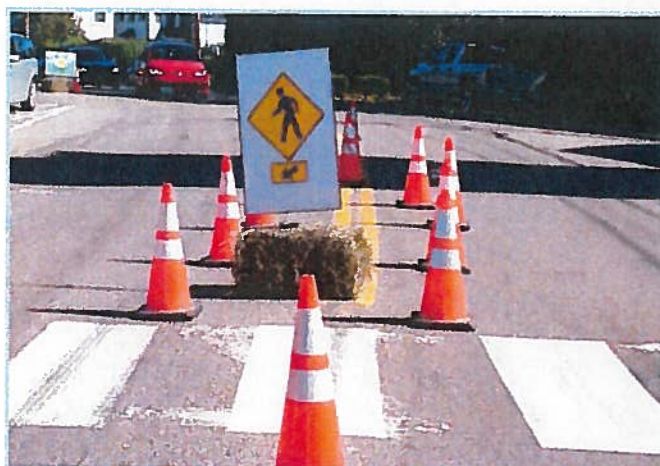
Improve pedestrian safety at crosswalks: Cones and a hay bale create a median refuge island, calming traffic and allowing pedestrians to cross the street in two stages
