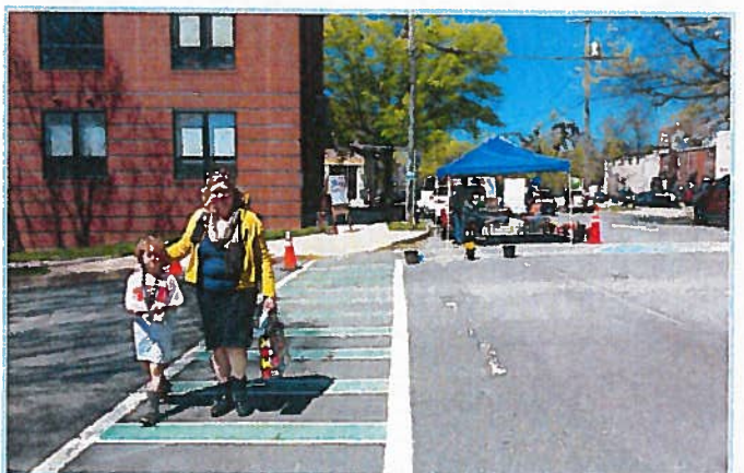
Increase the visibility of people crossing the street: Colored crosswalks and curb extensions delineated with cones and small plants enhance the pedestrian experience and shorten the crossing distance at this intersection.
