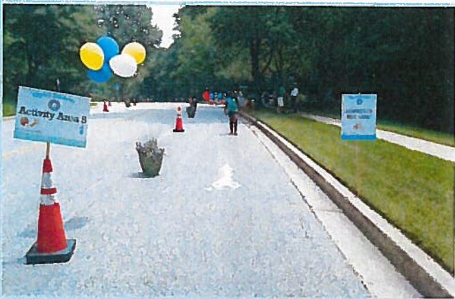
Create a comfortable bicycle facility: This demonstration of a separated bike lane reallocated an entire travel lane for bicyclists and pedestrians, and separated them from motor vehicle traffic with cones and planters.
